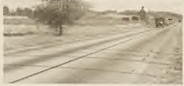
FIGURE 12.—SPEEDMETER AND PLACEMENT DETECTORS INSTALLED ON A TWO-LANE ROAD.
